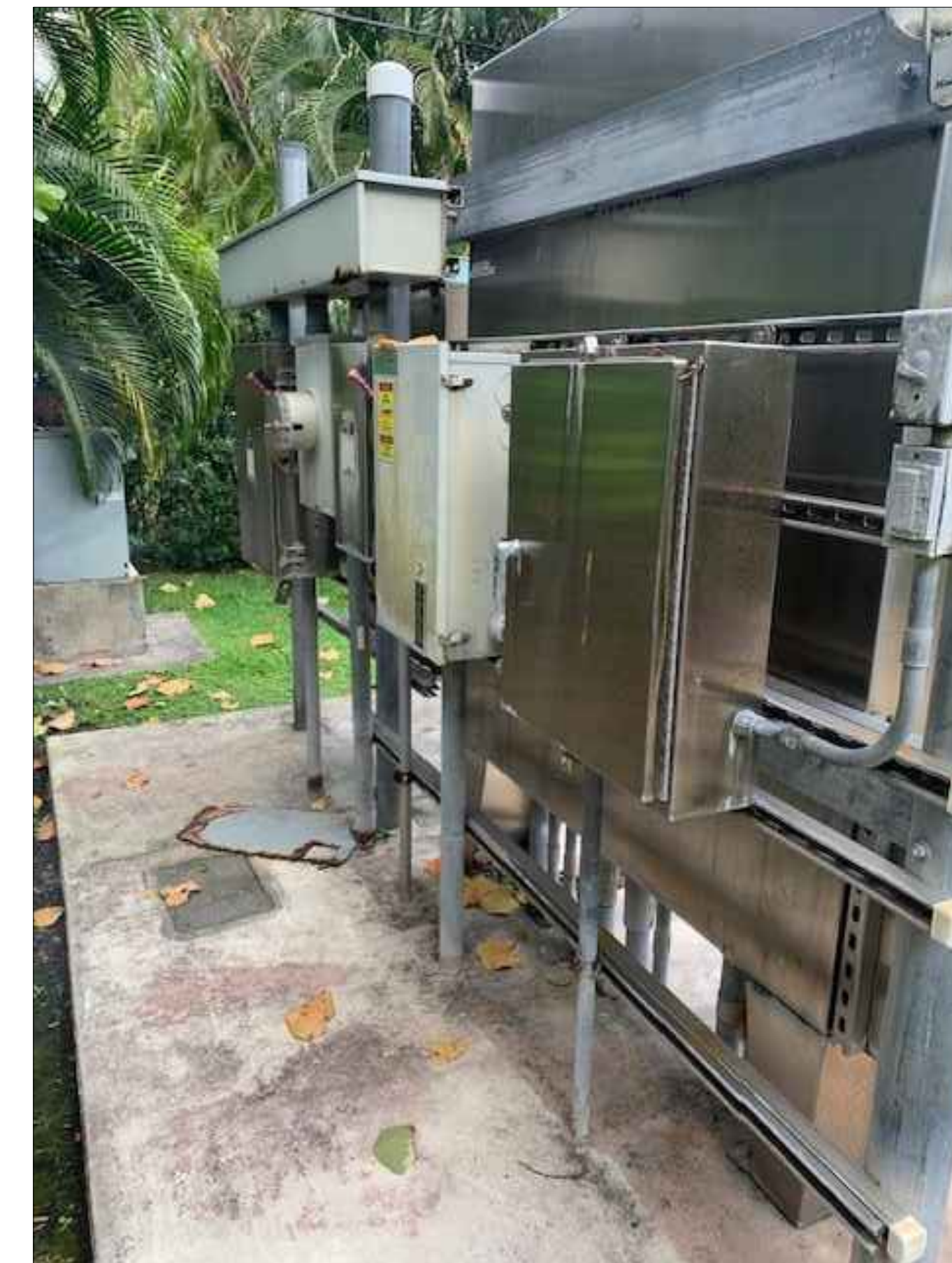
EXISTING UNI-STRUT RACK NTS
